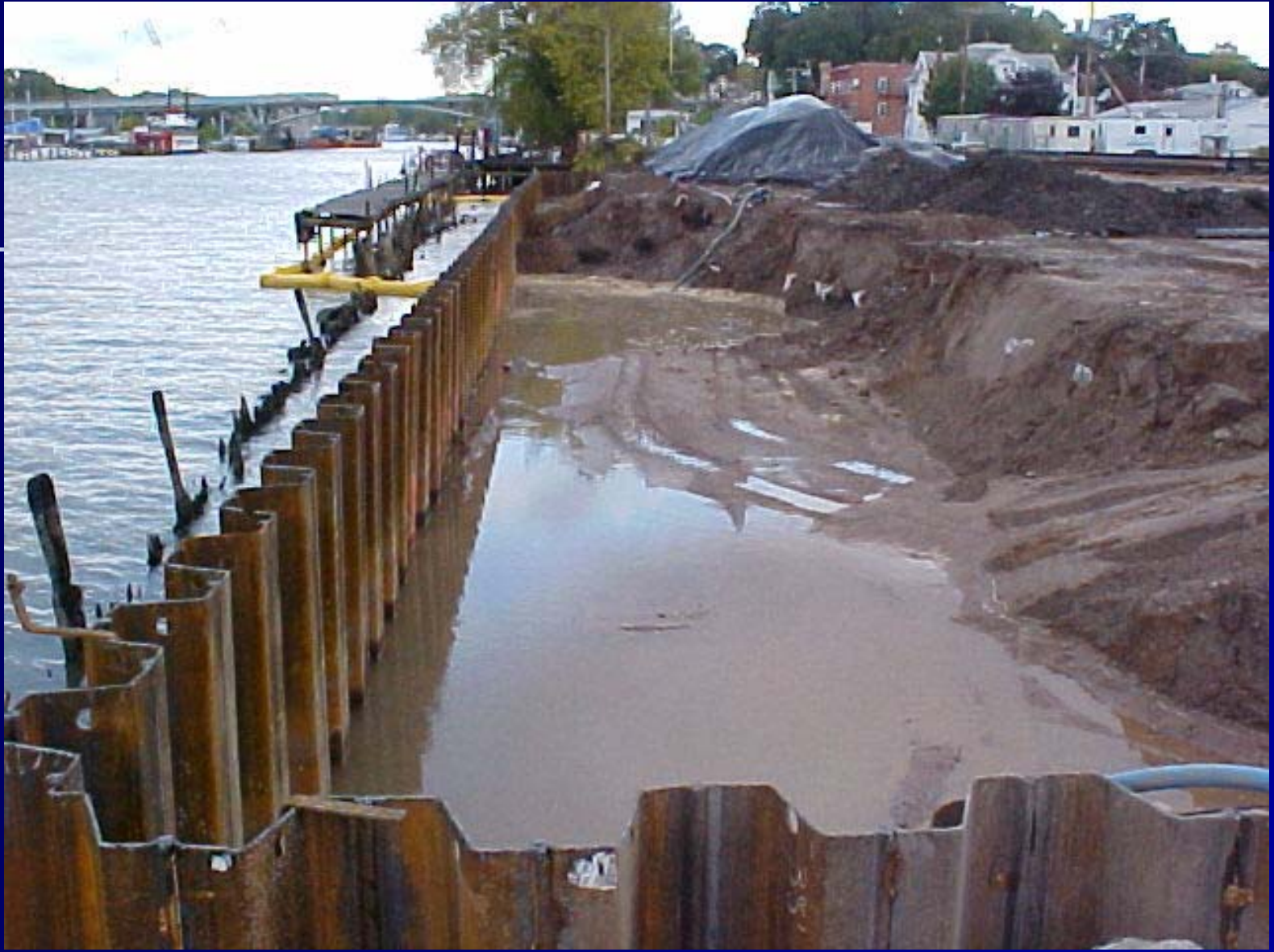
CSXT IRM Riverbank Excavation: October 2003
